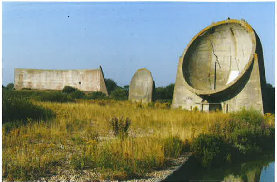
The Sound Mirrors - 200ft wall, 20ft dish and 30ft dish.
